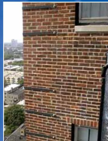
*Masonry corners are particularly susceptible to instability when a wall is in distress. Steel straps are used to keep the corner in place until demolition can begin.*
