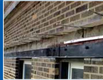
*One common method for supporting brick is to install stainless steel rods*
