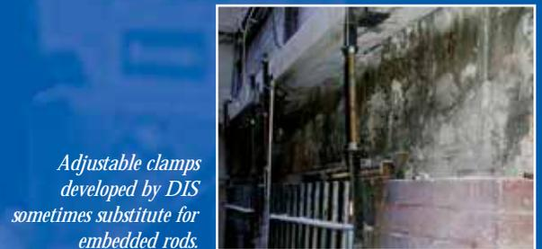
*Adjustable clamps developed by DIS sometimes substitute for embedded rods.*
