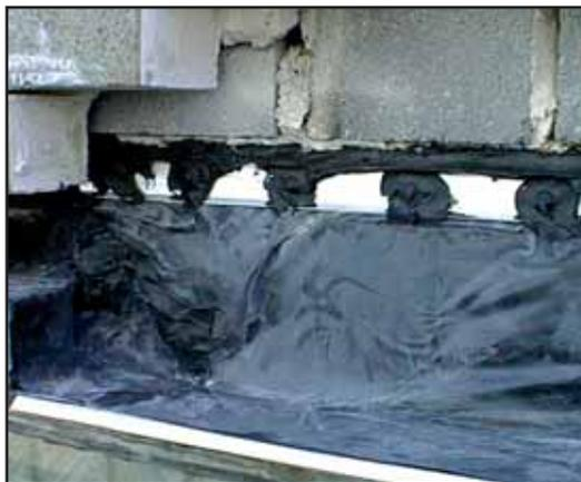
Prior to beginning any work, the masonry above the steel must be stabilized and supported, (see Structural Elements in this issue). With supports in place, the existing angle is replaced, the new steel is primed and painted then bolted into place. Flashing is placed over the angle so that any water entering the wall system will be directed out. The new brick placed on this flashing will have weeps placed at the flashing to allow trapped moisture to flow freely out of the wall cavity.
