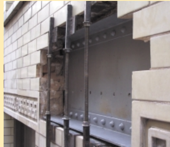
Above: Bracing support system at 28 East Jackson
